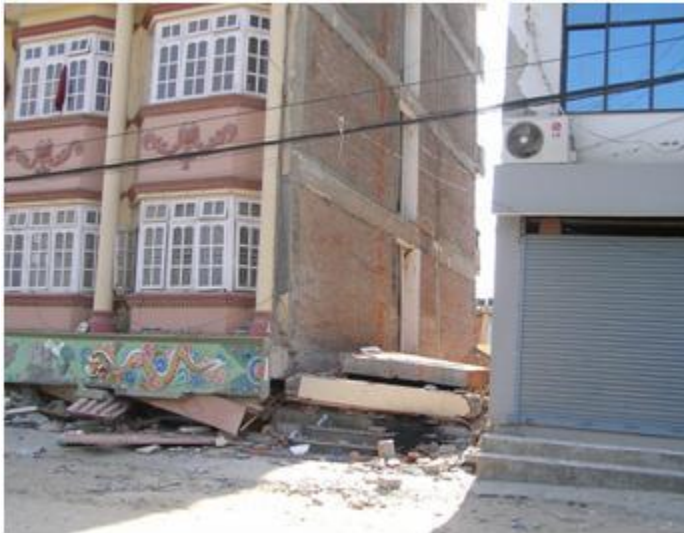
Fig. 2- Open ground storey failure of 5 storey building, Kathmandu during the 2015 Nepal Earthquake
