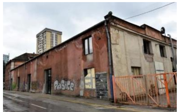
Fig 3:- Abandoned Steel factory, Vaso Miskin Crni (Source: klix.ba)
