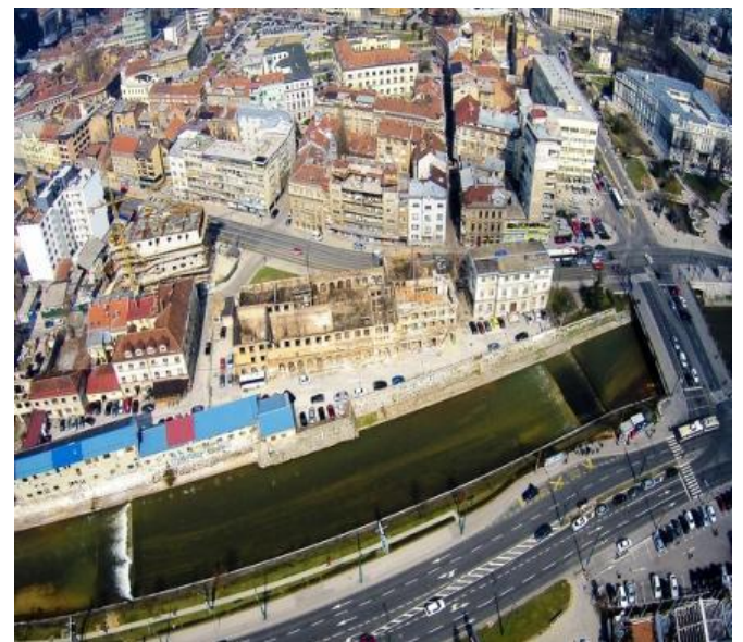
Fig 34:- Aerial Photo of Electrical Power Station and Surrounding, 2017 (Source: m-kvadrat.ba)
