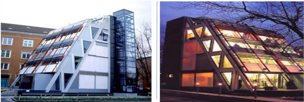
Fig 4:- The Swiss composite LED (light emitting diode) glazing façade - source : *Swissbau et al. (2007)*
