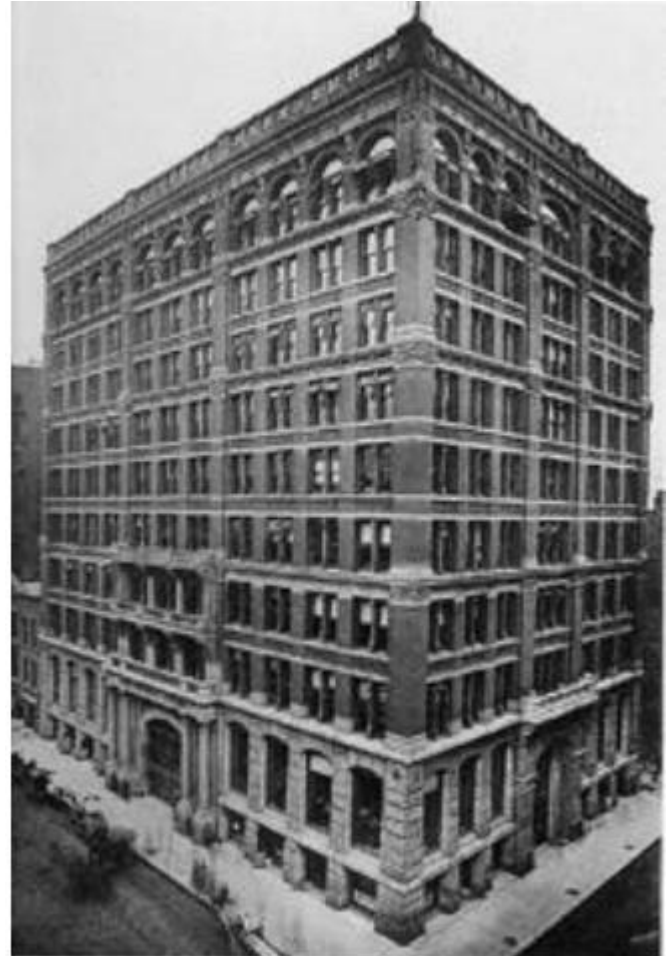
Fig 1:- Insurance Building, Chicago, USA, 1885
