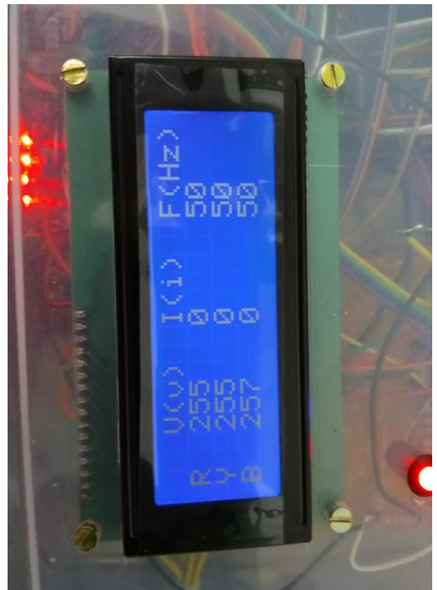
Fig 13:- Measuring runtime values for a 3-phase system without load
