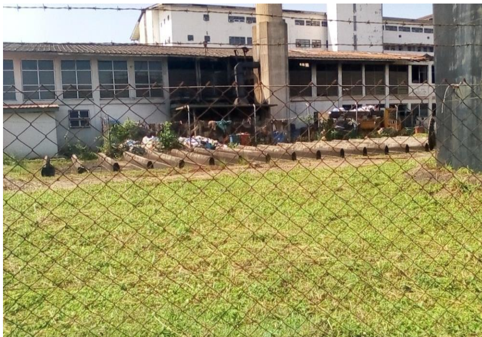
Fig 3:- A Placed assumed to be Waste Storage Plant with Garbage Truck in Front
