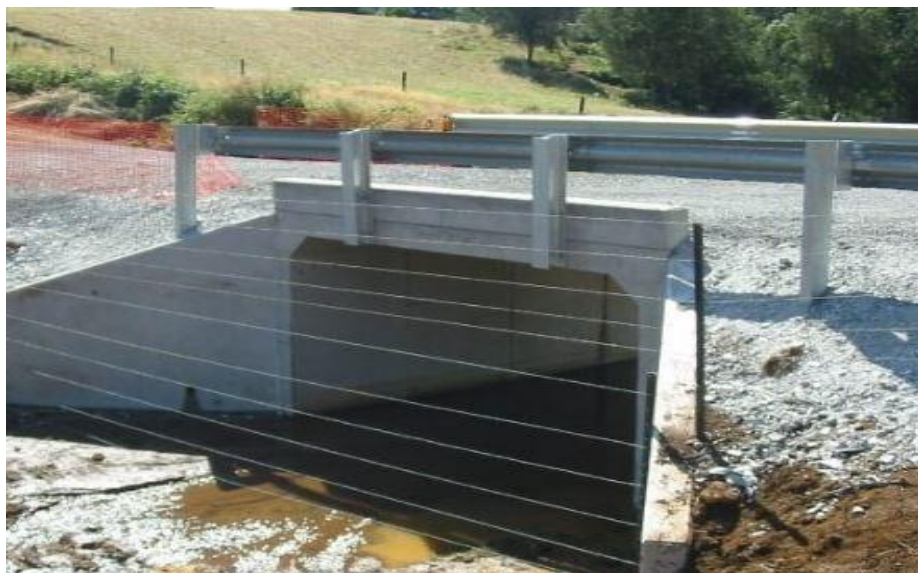
Fig 8: Rcc Solid Slap Culvert with a filter
