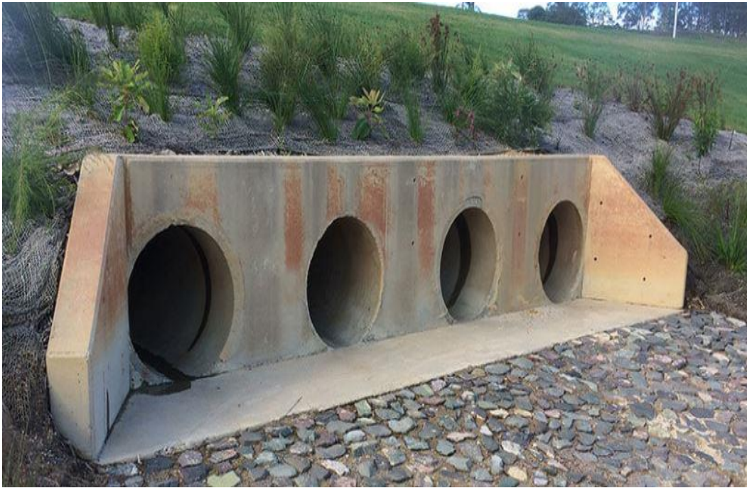
Fig 1:- Pipe Culvert
