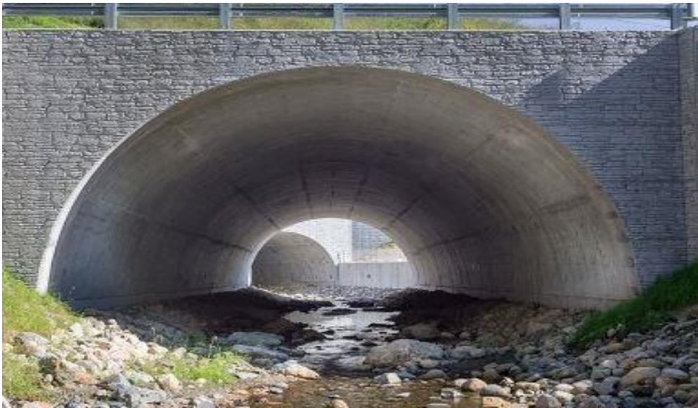
Fig 5:- Pipe Arch Culverts
