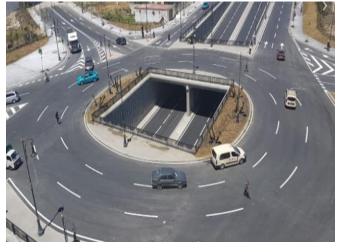
Fig. 1. Roundabout with underground passageway
