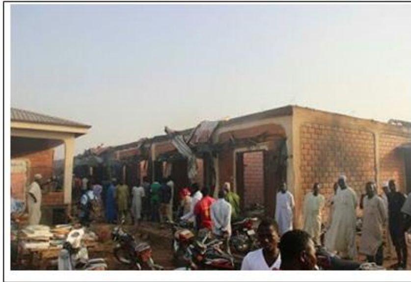
Fig 10:- Engr. Abdulkadir Abdullahi Kure Ultra-Modern Market Roofs After External Fire Spreading
