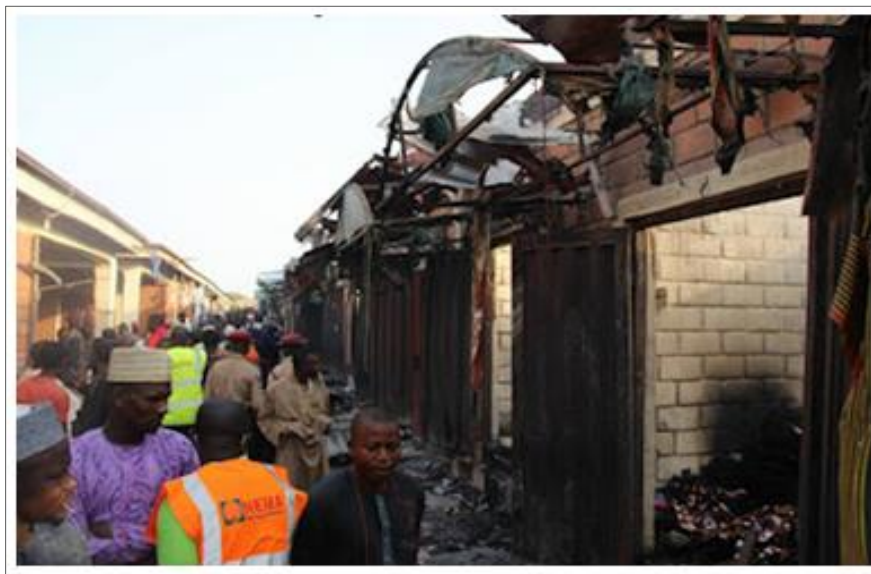
Fig 9:- Engr. Abdulkadir Abdullahi Kure Ultra-Modern Market Shops Doors After External Fire Spreading [16]
