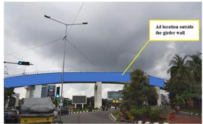
Fig 3:- Advertisement Location in the outside crossing wall of rail
