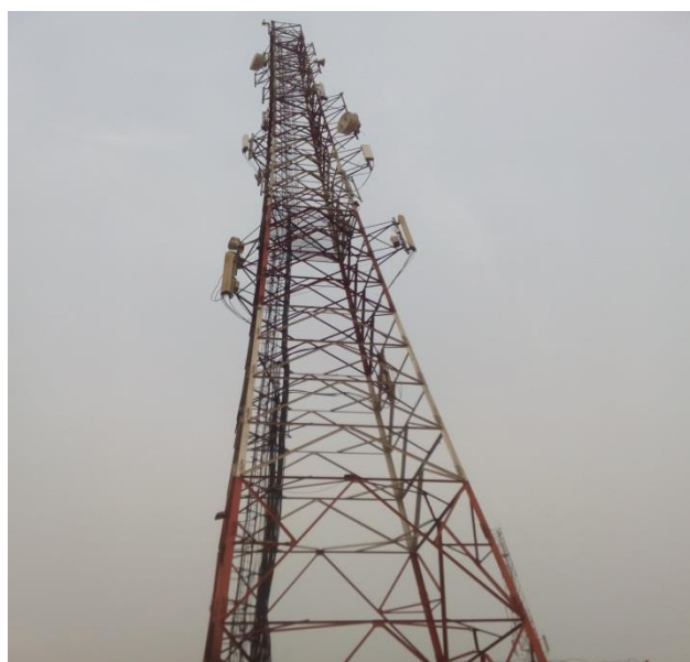
Fig 1:- Typical macro base station
