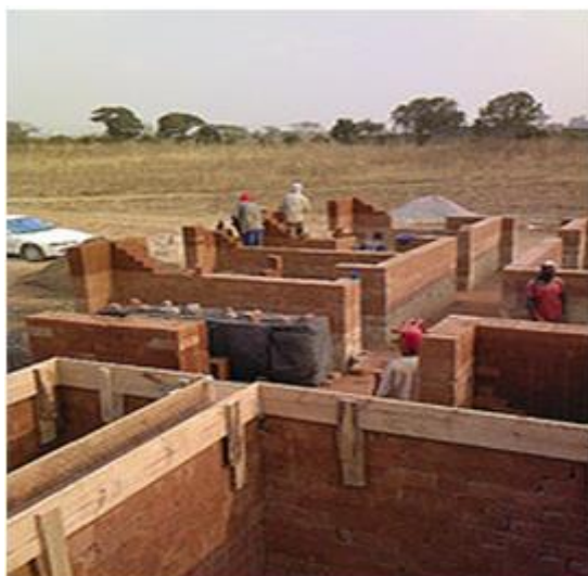
Fig 2:- House under construction in Zambia
