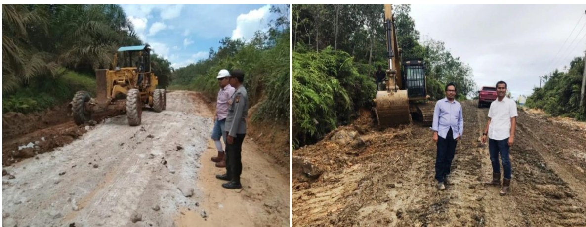
Fig.4.Site Condition on The Maluku Bantanan Road
