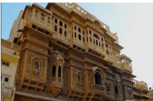
Figure 3 Textured wall and Jharokha with Jalli detail on Patwon Ki Haveli, Jaipur
