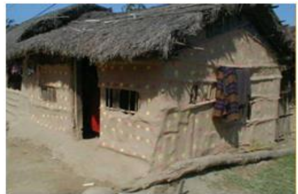
Figure 4 Shading device and small window detail from a kacha house in Rajasthan
