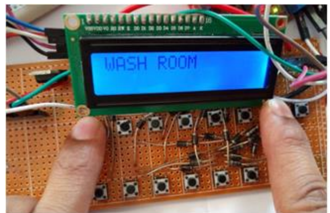
Fig. 8: "WASH ROOM" Displayed when switch-16 & 10 are pressed.
