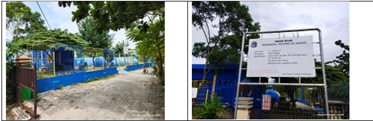
Fig. 5: Waste water treatment plant facilities at Tidung Besar Island
