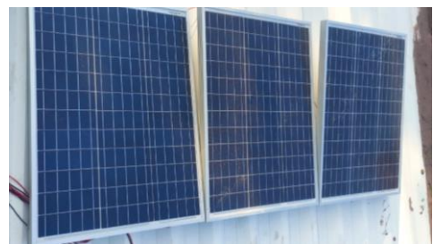
Fig. 2. The process of installing polycrystalline solar panels on the housetop
