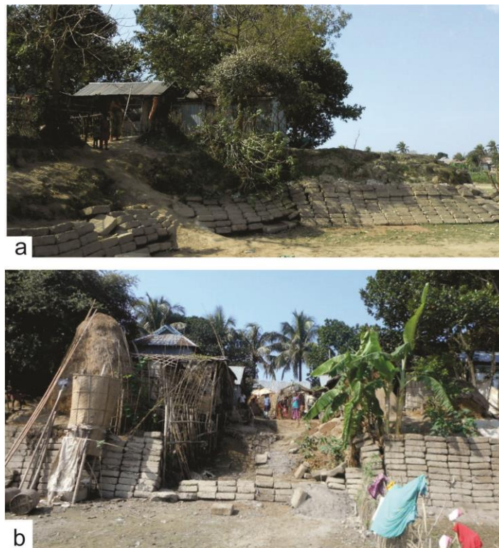
Fig. 5: Varying states of concrete block revetment walls around the Concernpara settlement. (Field survey, 2016 and 2021)
