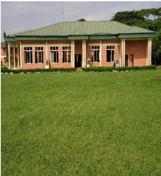
Plates 3: Image showing purpose-built, building envelope openings in the Edozien Lecture Theatre Source: Author's Fieldwork, 2022
