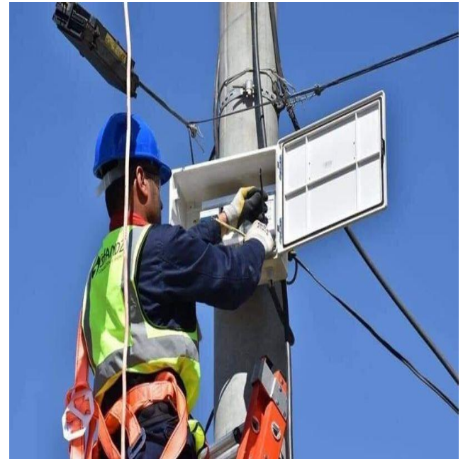
Fig . 2 / smart meter installation
