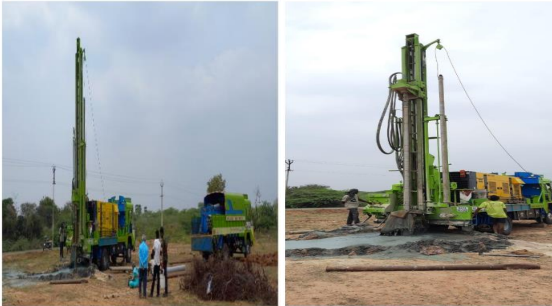
Fig. 11: Bore hole drilling
