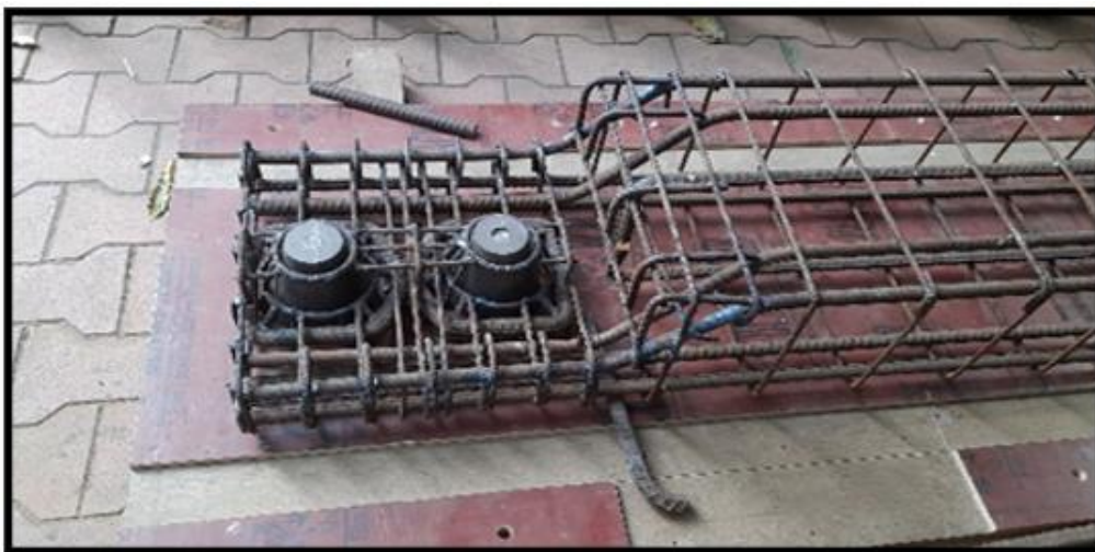
FIG 17: COLUMN CONNECTION CAGE
