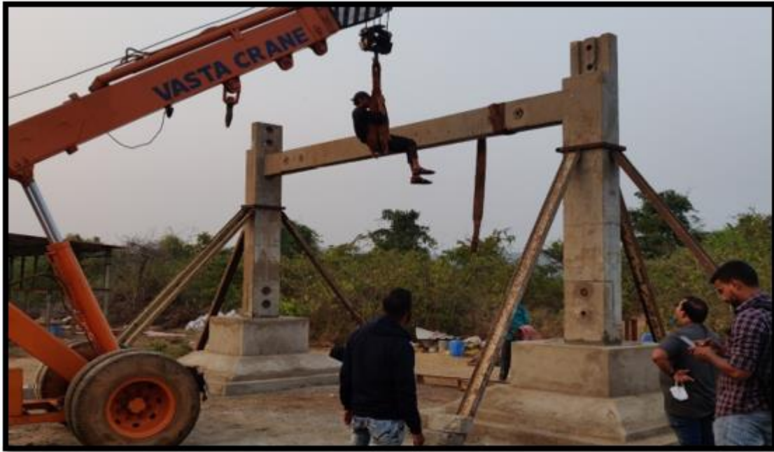
FIG 22: ASSEMBLY OF FRAME IN PROGRESS.
