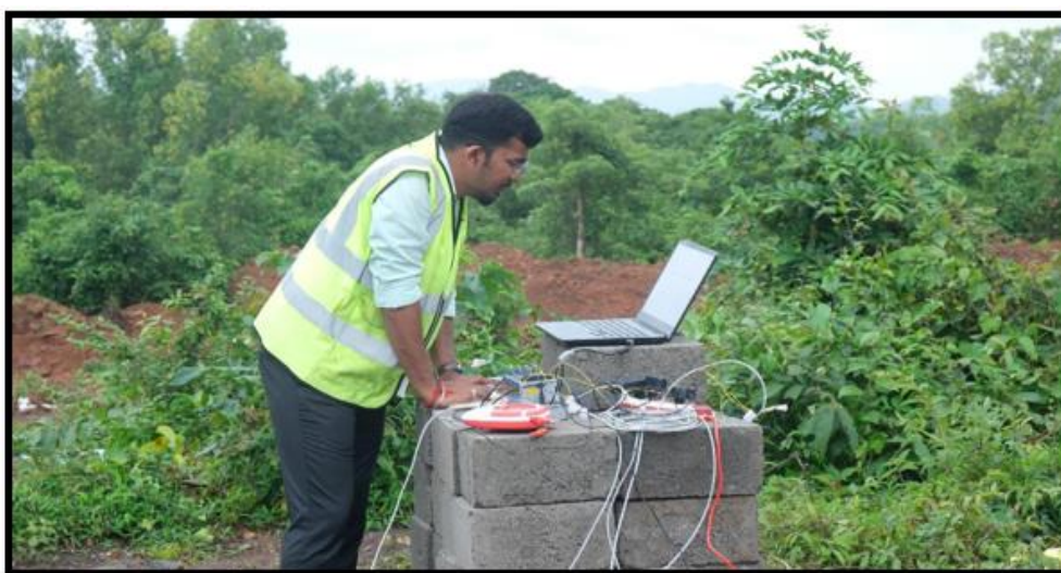
FIG 54: DATA ACQUISITION – SET UP
