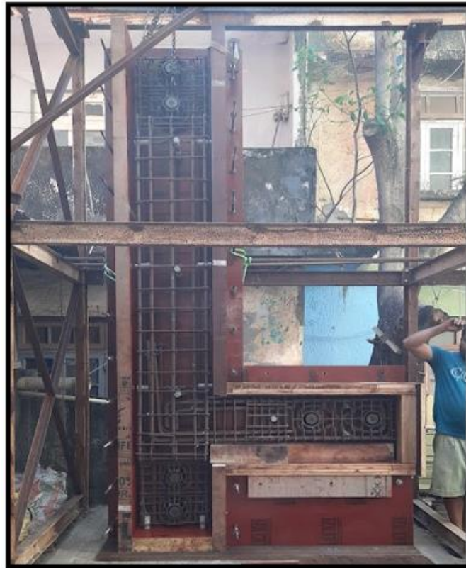
FIG 18: REINFORCEMENT IN WOODEN SHUTTERING.
