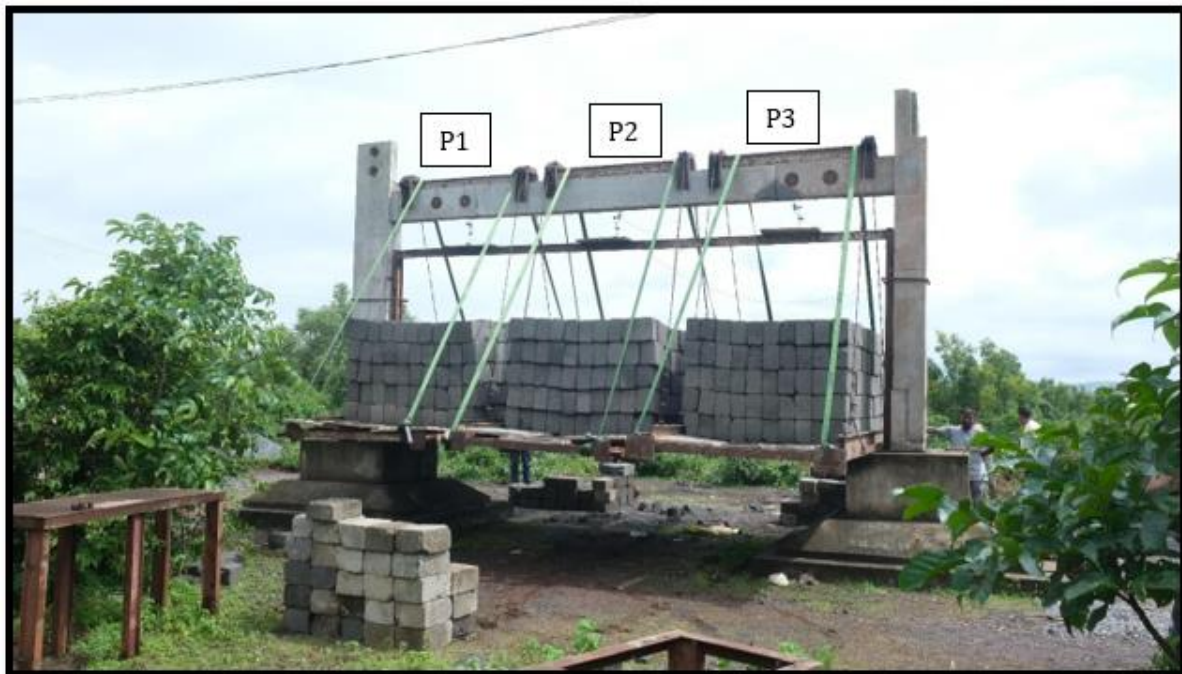
FIG 56: FULLY LOADED SUSPENDED PLATFORM
