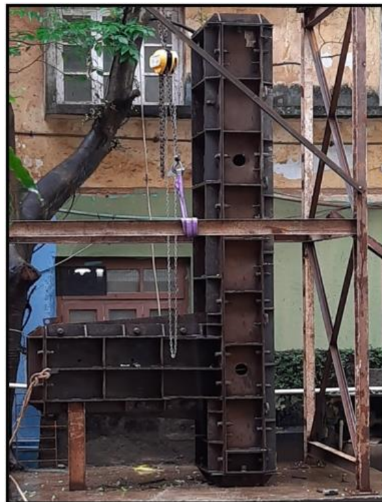
FIG 19: STEEL SHUTTERING.
