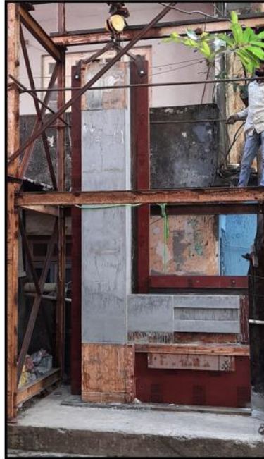
FIG 20: COLUMN AFTER DE-SHUTTERING.
