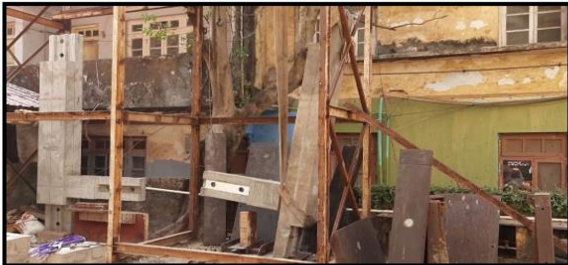
FIG 21: COLUMNS AFTER DE-SHUTTERING, READY FOR TRANSPORTATION
