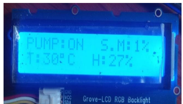
Fig 17 Water Pump ON
