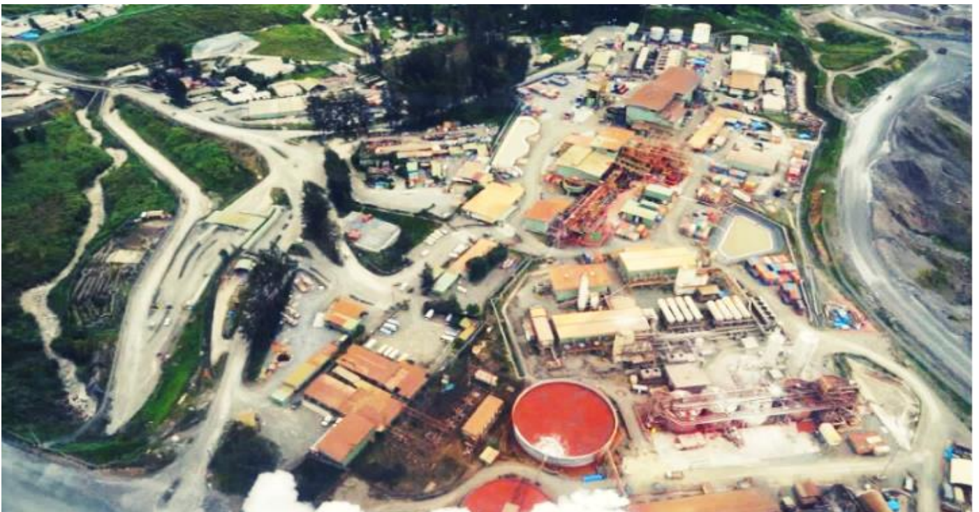
Fig 3 Mill and administration facilities within the SML (Source: PJV)
