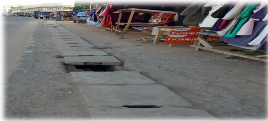
Plate 2: Street closed drainage channel
