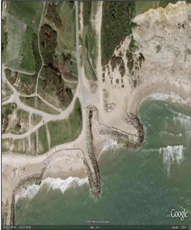
Plate 3. Culvert between Groynes at outlet of Chewton Bunny (Satellite image: Google Earth, 2008)
