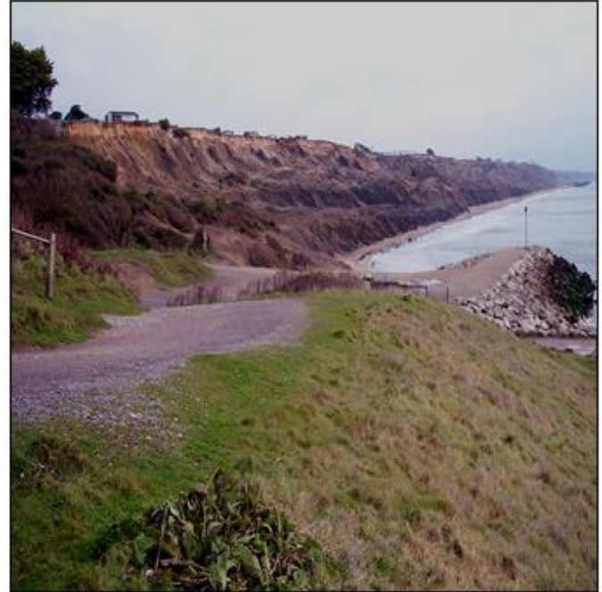
Plate 4. Slumping cliffs at Barton-On-Sea (Photo: M. Hackett, 2008)
