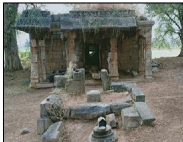
Fig 2 Collapsed Front Mandapam of 'Adi Narayanaperumal' Temple
