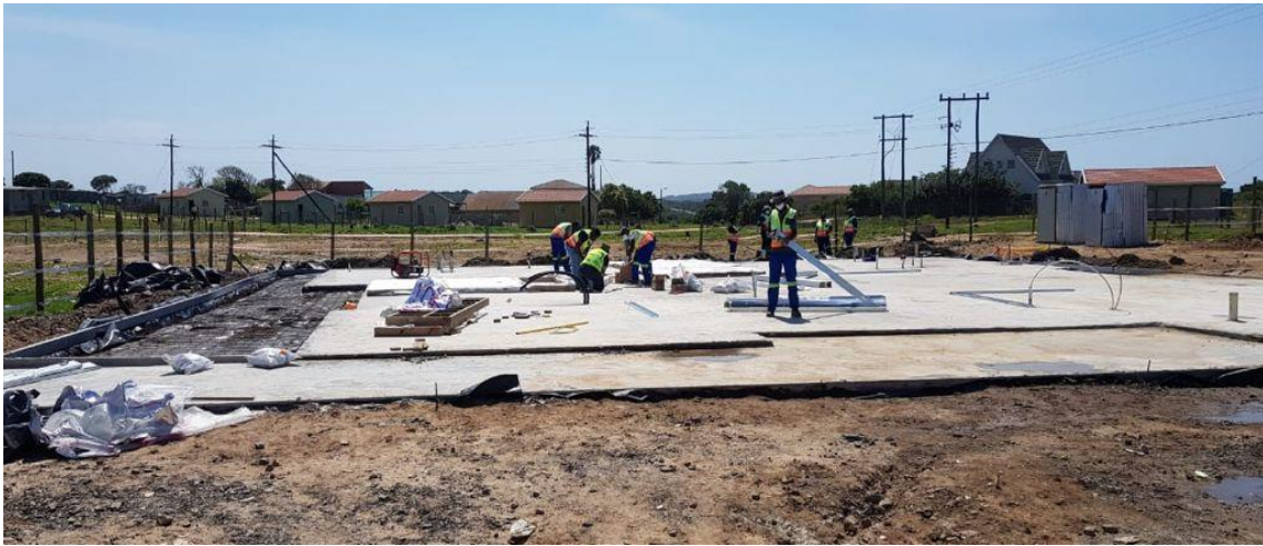
Fig. 4: Eco- Village Site Construction (Source, own), 2020
