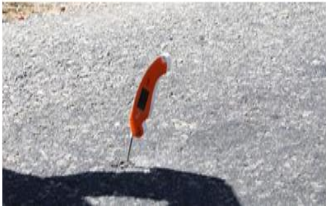
Fig 4 Measurement of Pavement Temperature
