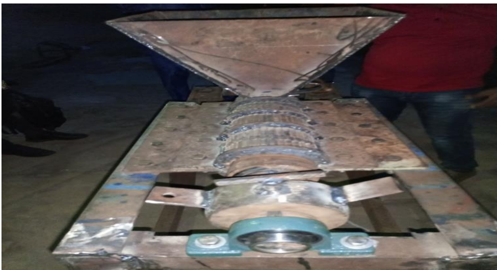
Fig. 19: Pictorial view of the bearing, adjustable cone and barrel during construction
