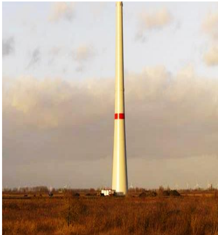
Fig 5 Tubular Steel Tower
