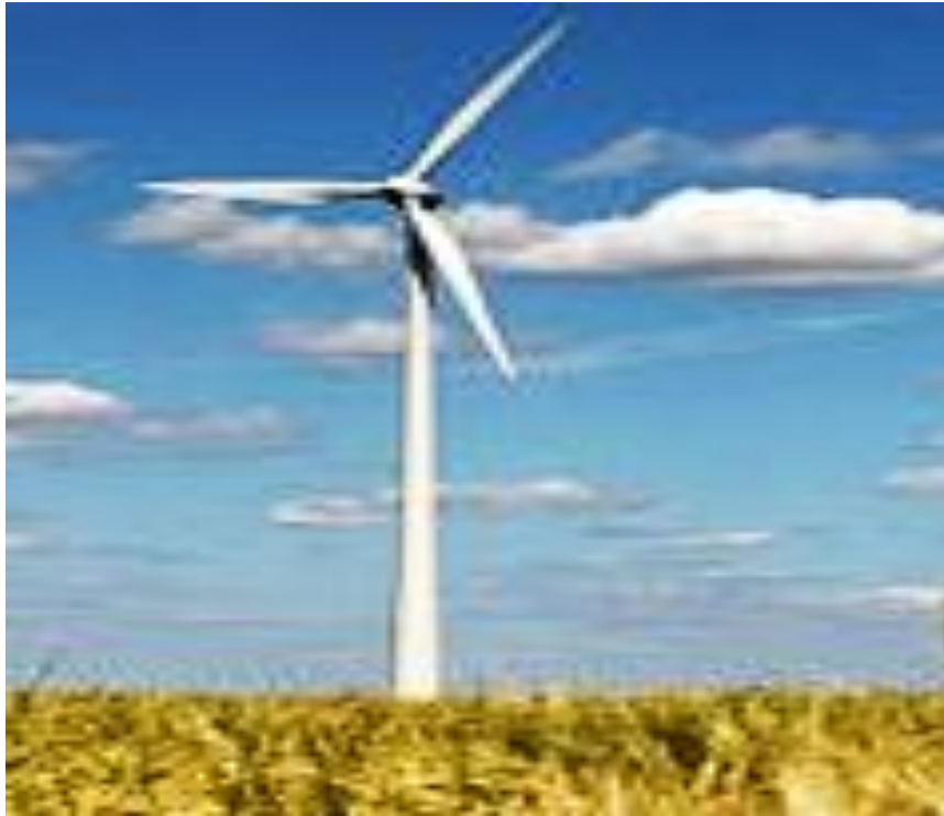
Fig 2 Horizontal Wind Turbine
