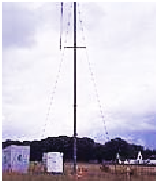
Fig 7 Guyed Pole Tower
