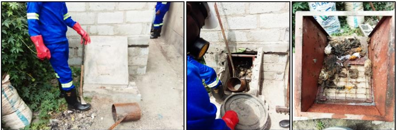
Fig 10: L-R, Opening and Removing Solid Waste from the Trash Chamber
