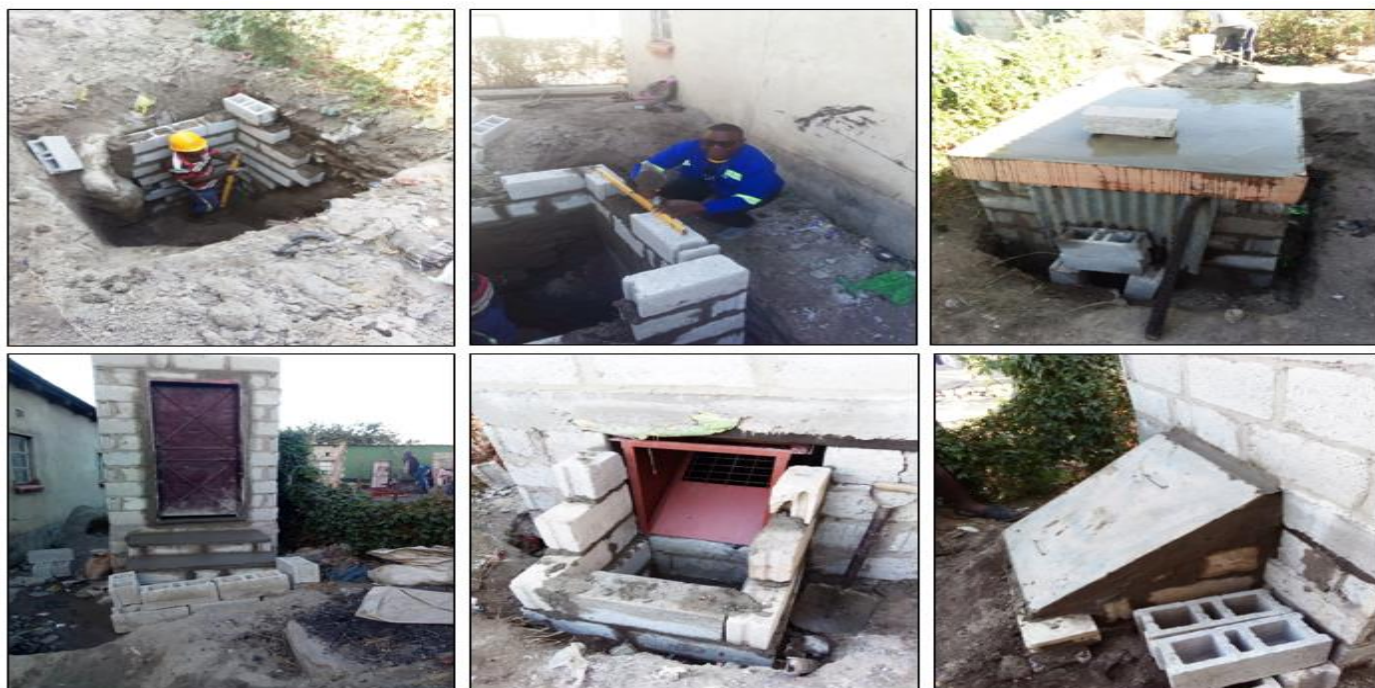
Fig 12: Stages of the Pit Latrine's Construction
