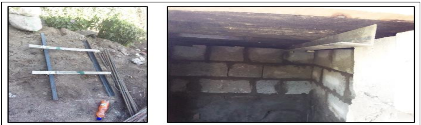
Fig 9: Angle Bar Supports Beneath the Slab
