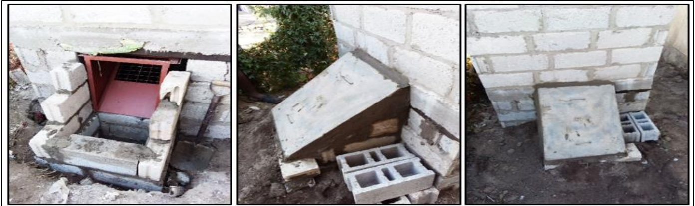
Fig 8: L-R: Construction of the Trash Chamber
