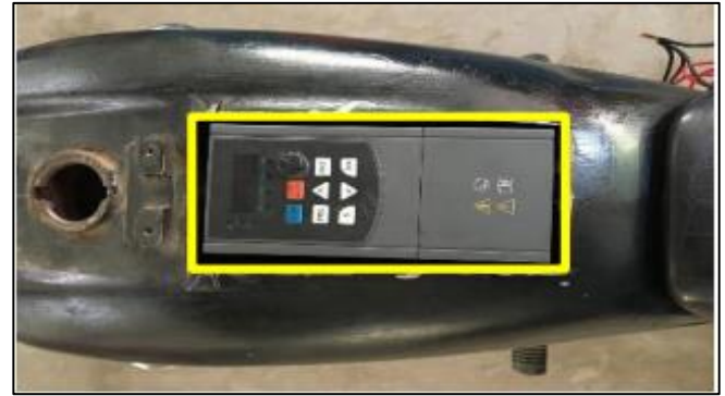
Fig 5 VFD Placed in Fuel Tank
