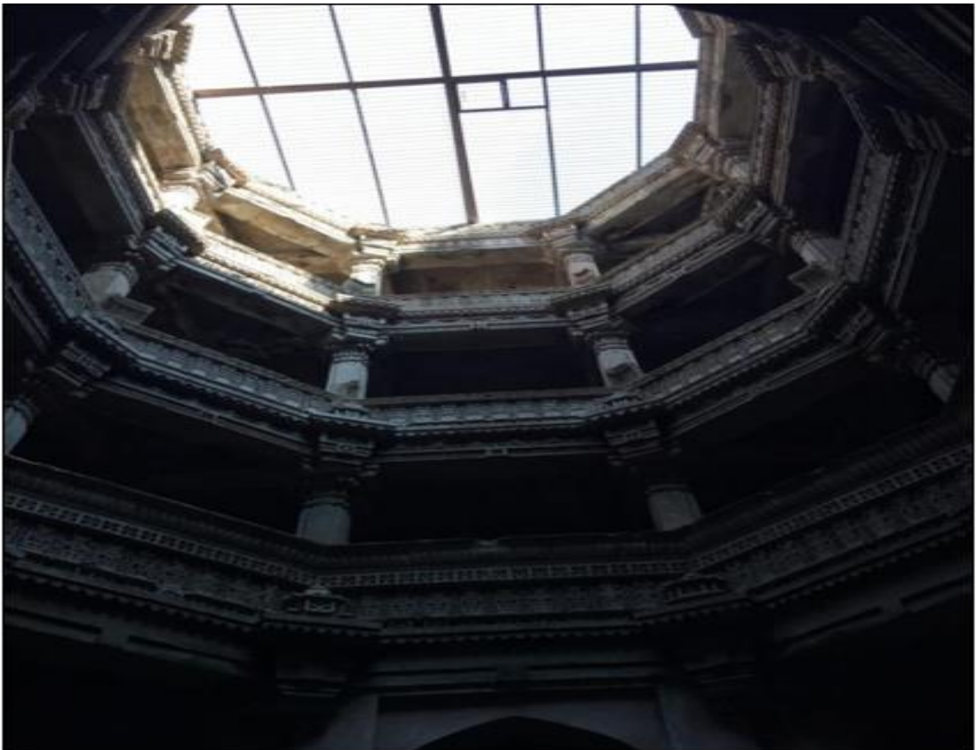
Fig 10 Covering at the Top of the Structure to Protect the well
