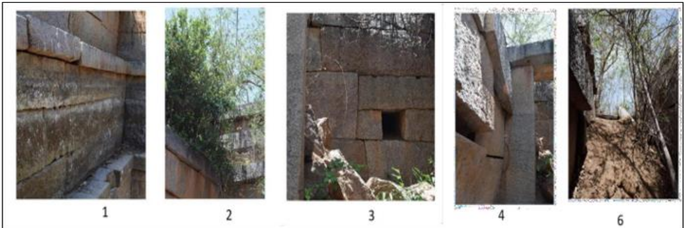
Fig 25 Existing Condition of Step Well Source: Primary Survey
