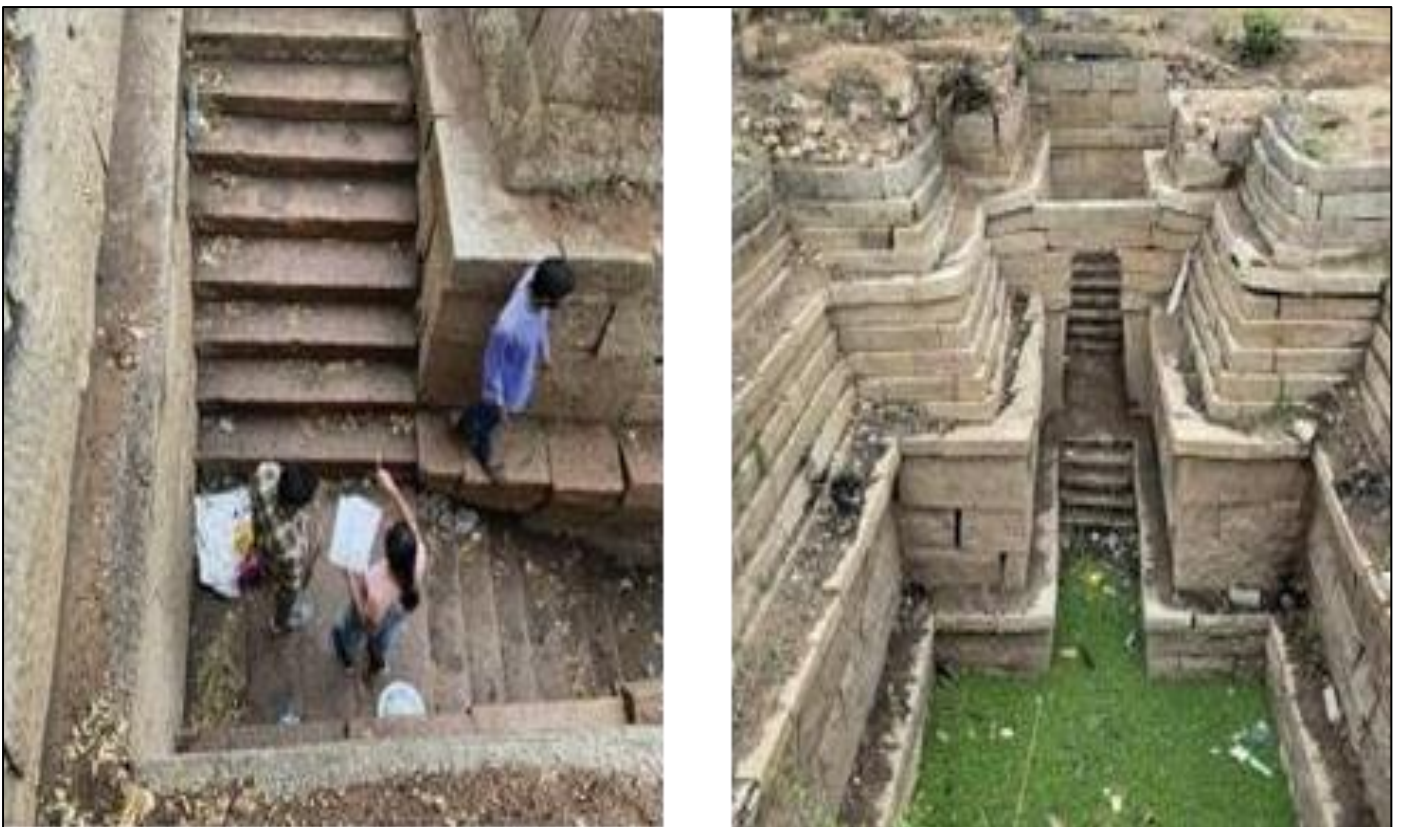
Fig 19 Existing Condition of Step Well Source: Primary Survey
