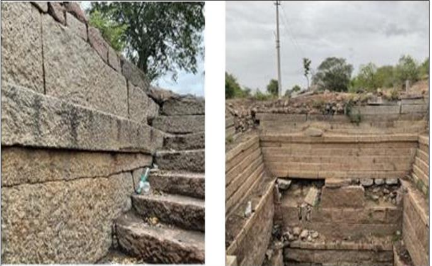
Fig 18 Existing Condition of Step Well Source: Primary Survey
