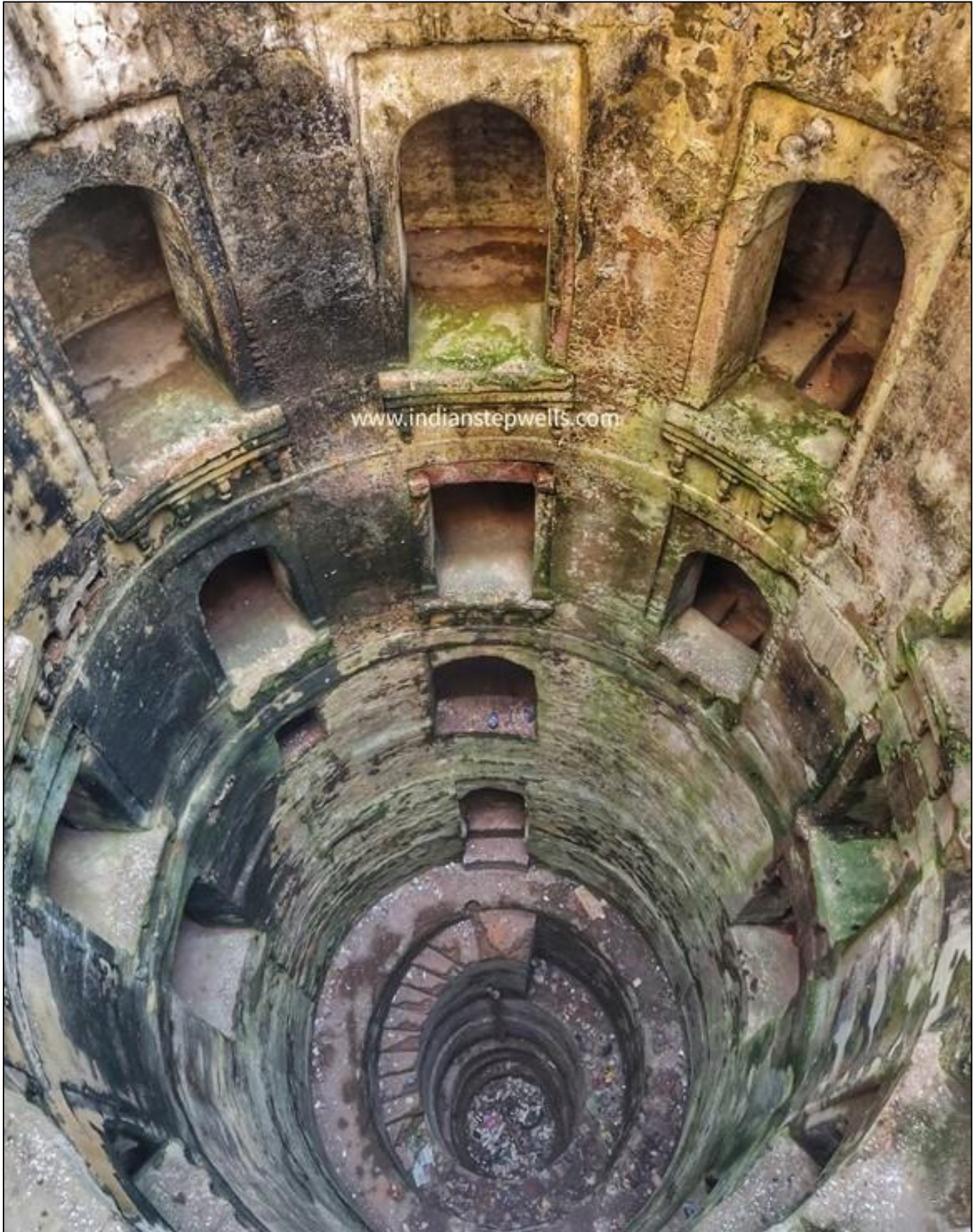
Fig 5 Halisa Stepwell - Badra Type at Gujarat Source: Indian Step Wells
