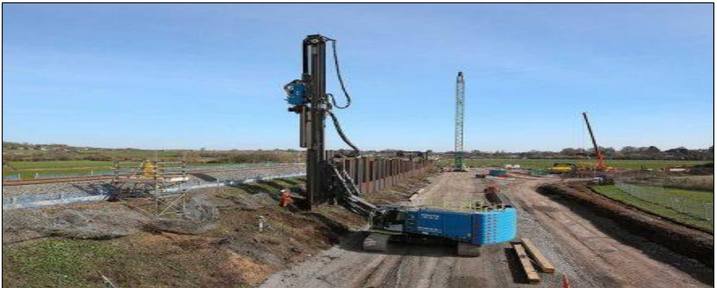
Fig 15: Somerset Railway Embankment Stabilized Using Sheet Pile Walls (geplus.co.uk 2021)
