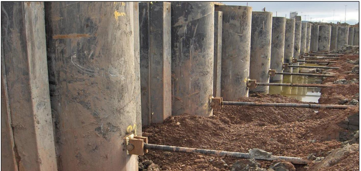
Fig 17: Anchoring System of Sheet Pile Walls Courtesy of db-excel.com, (2017)
