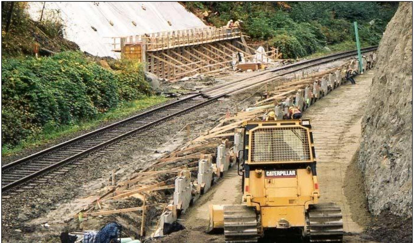
Fig 6: MSE Walls Used As Railway Retaining System-Courtesy of Charley Chambers (AREMA 2023)
