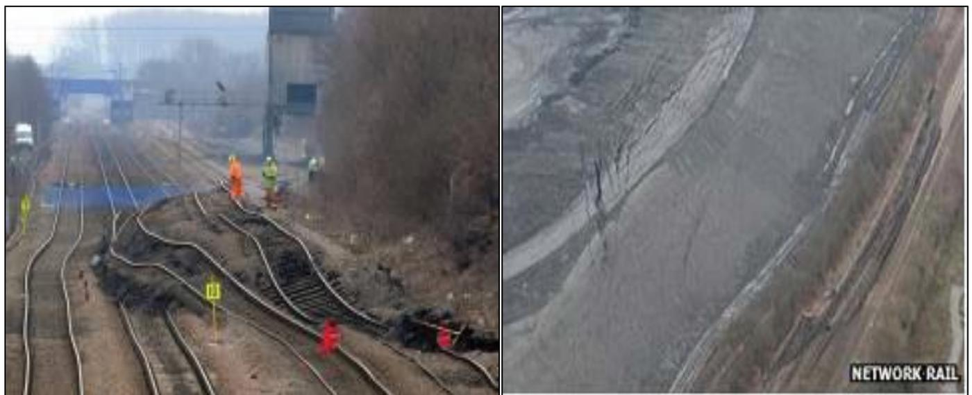
Fig 25: Landslip Rail Line in UK, February 2013: View of the Railway (Left); Top View of the Area (Right). (Clemente Fuggini et al 2016)
