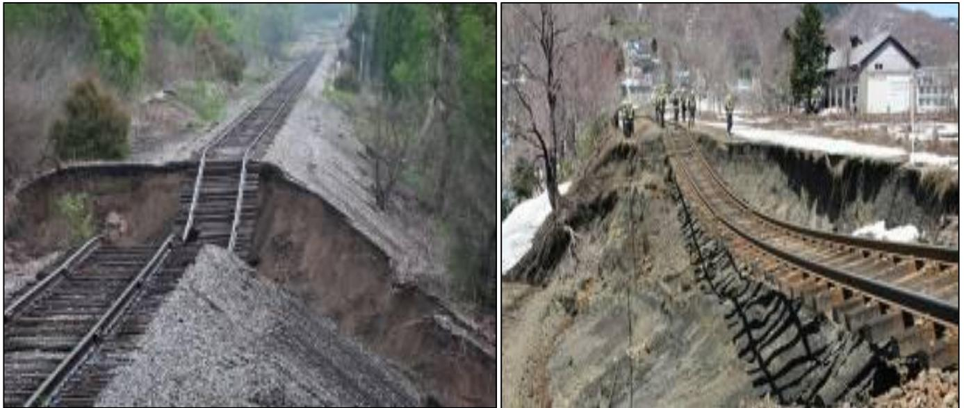
Fig 24: Collapse of Railway Embankment along Plymouth Rd, Ann Arbor, US, in May 2011 after an Heavy Rain on Already Saturated Ground (Left); Massive Landslide in Hokkaido Leaves Railway Tracks Hanging in Mid-Air, April 2012 (Right). (Clemente Fuggini et al 2016)
