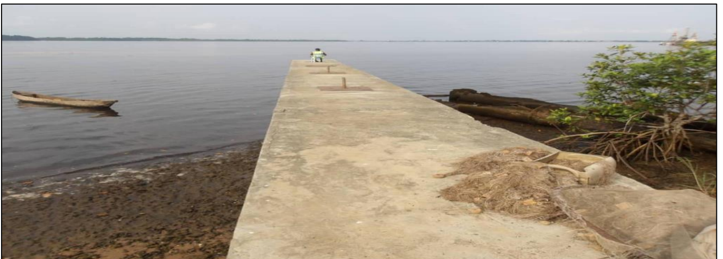
Image 6: Concrete spillway for Treated Effluent from SOCIR into the Congo River Source: Daniel Mudinga, 2023
