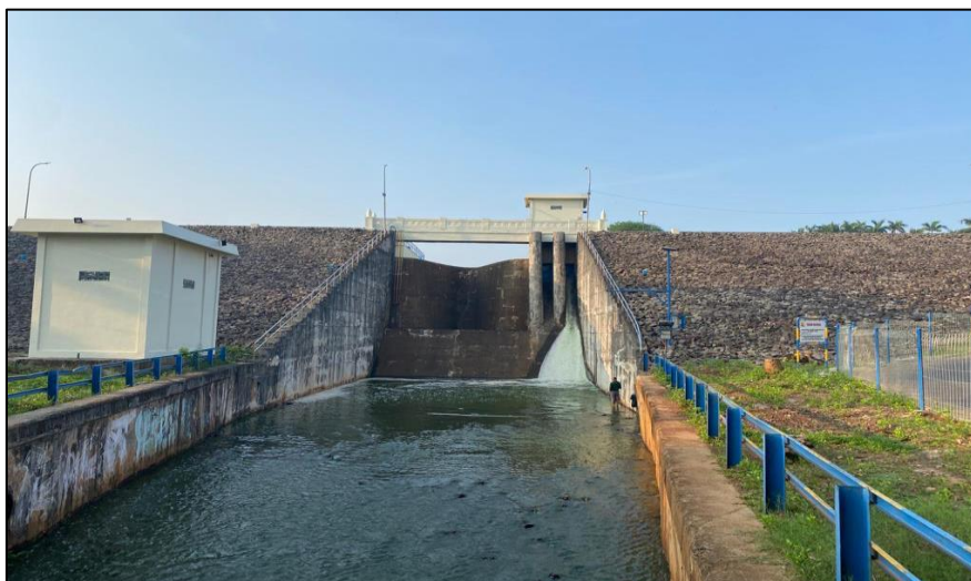
Fig 8 : Spillway of the New Dam, Source : Personal documentation July 2024.
