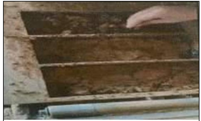
Fig 3: Filling the Mould with Wet Mixture
