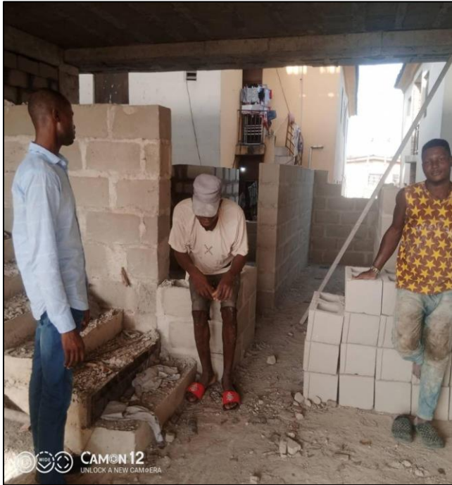
Fig 2: A Picture Showing an Interview with Construction Masons at Ikeja, Lagos
