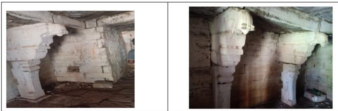
Picture 8 Joint Pillar Structure
