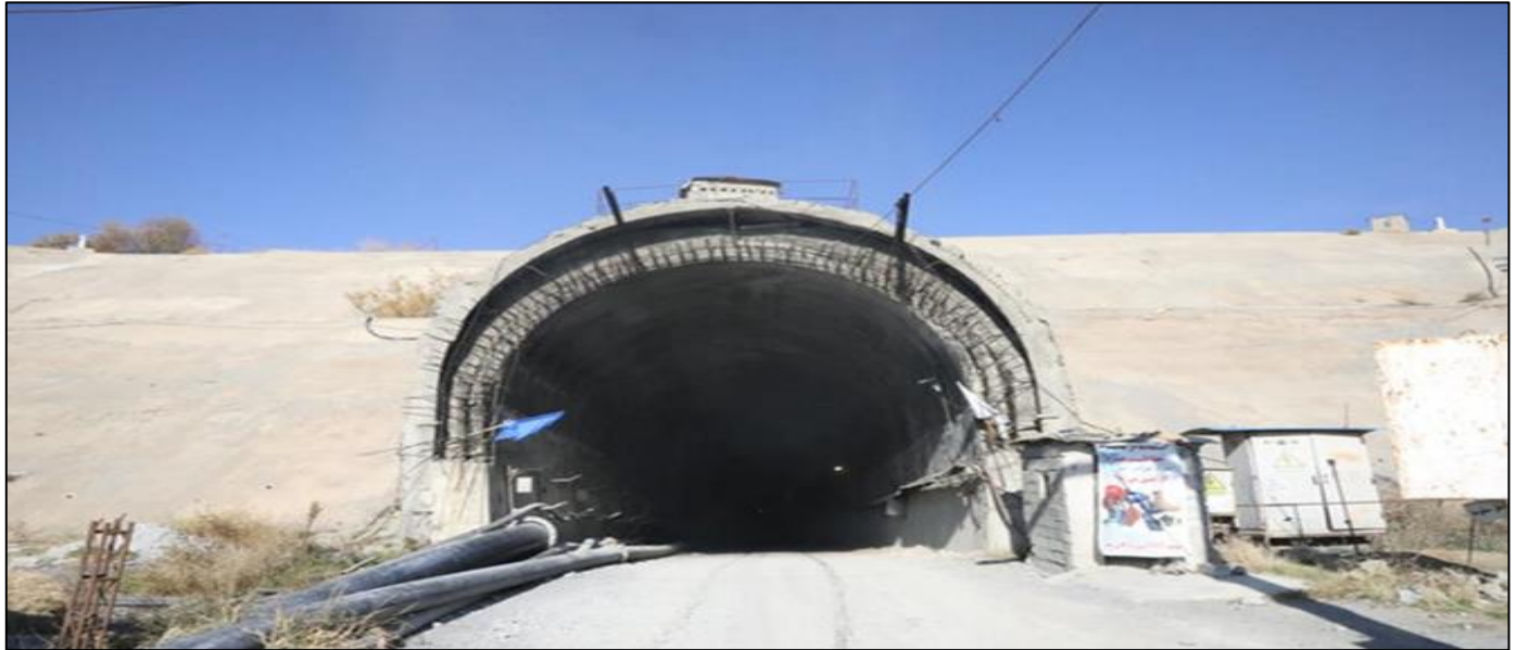
Fig 7: Construction of a Tunnel to Transfer Water to the Lake
