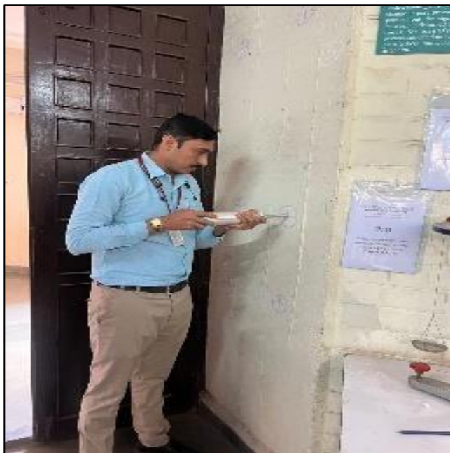
Fig 2: Our Project Guide While Testing on Structure with Rebound Hammer
