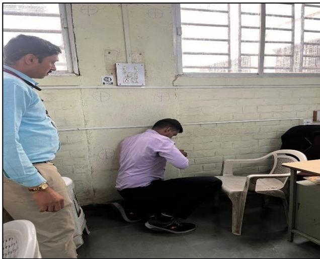
Fig 1: Photos while Testing on Structure with Rebound Hammer
