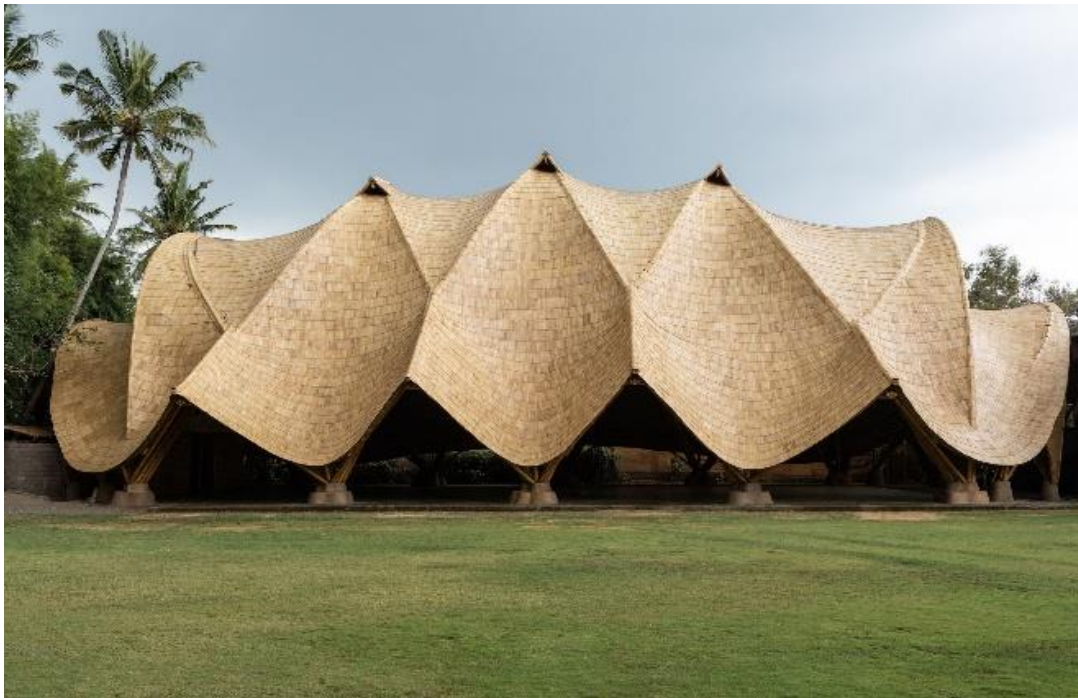
Fig 1. Green School in Bali, Indonesia (Johari, 2018).
