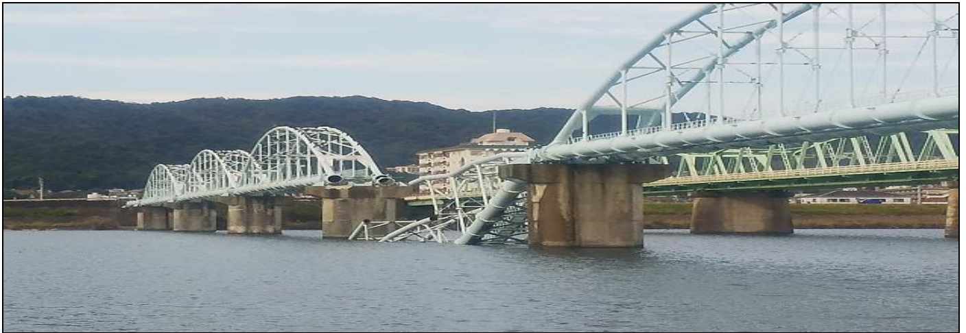
Fig 1 Wakayama Aqueduct Bridge Failure
