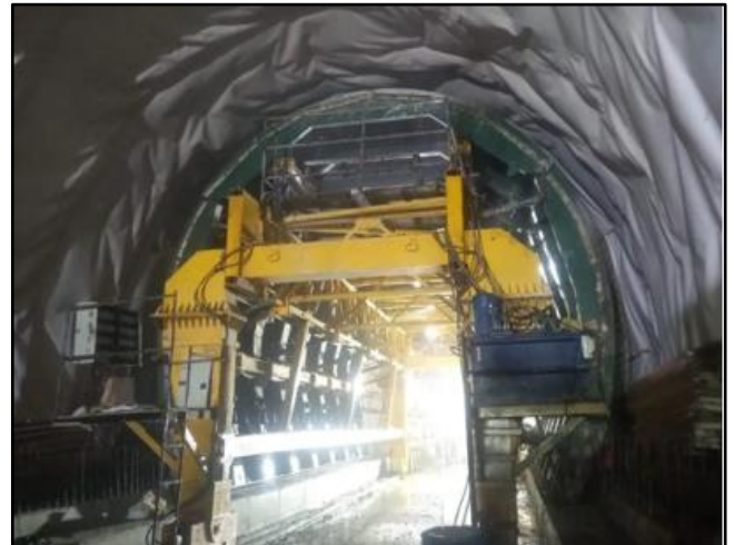
Fig 4 A Tunnel Lining Gantry Stationed at Hrishikesh-Karnprayag Rail Project Pkg 7b
