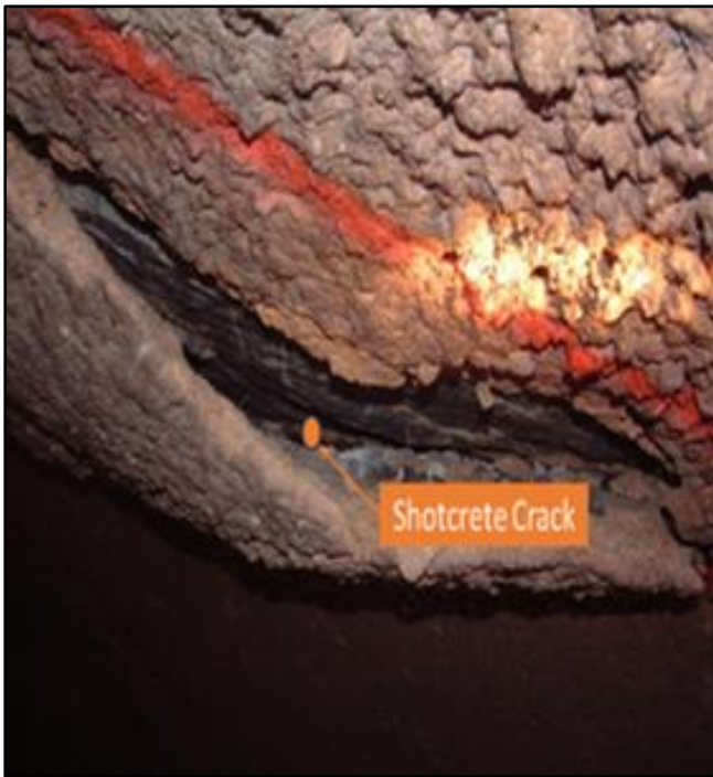
Fig 13 Typ. Overstressed Rock Mass
