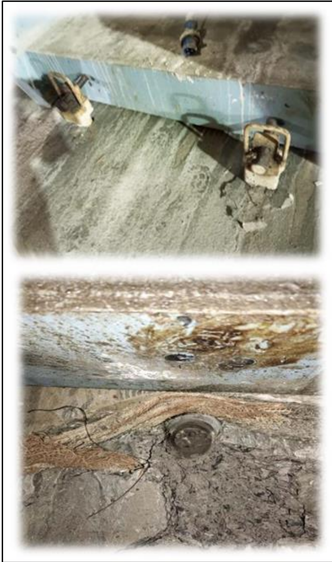
Fig 12 Highlighting Initial Cracks Observed in Kicker Beam (Top) & Spalling of Concrete After Removal of Pins (Bottom)
