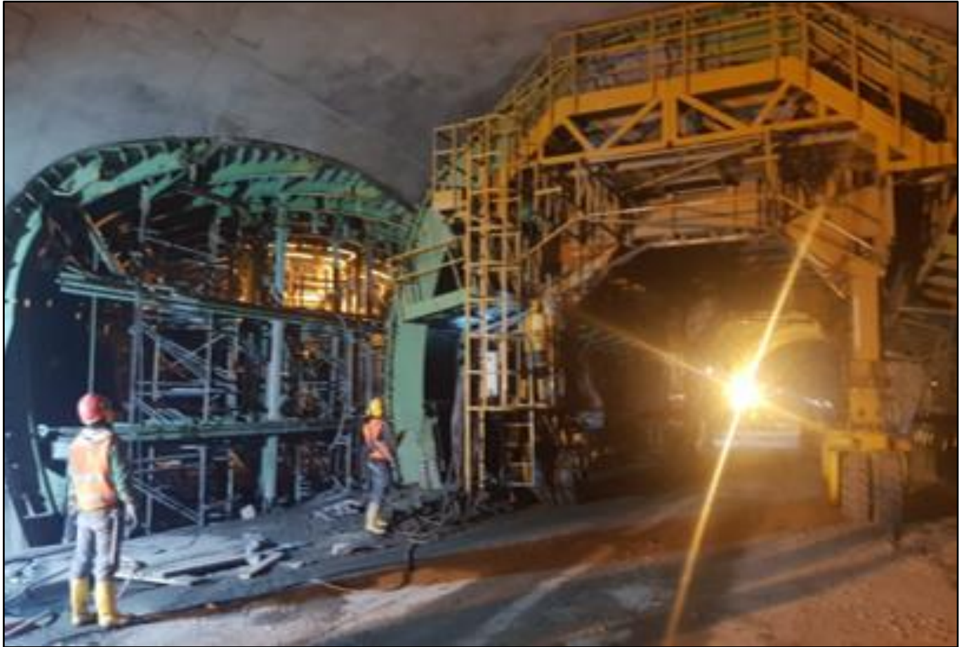
Fig 15 A Typ. Cross Passage Plug Formwork Fabricated by Rubrica Engineering
