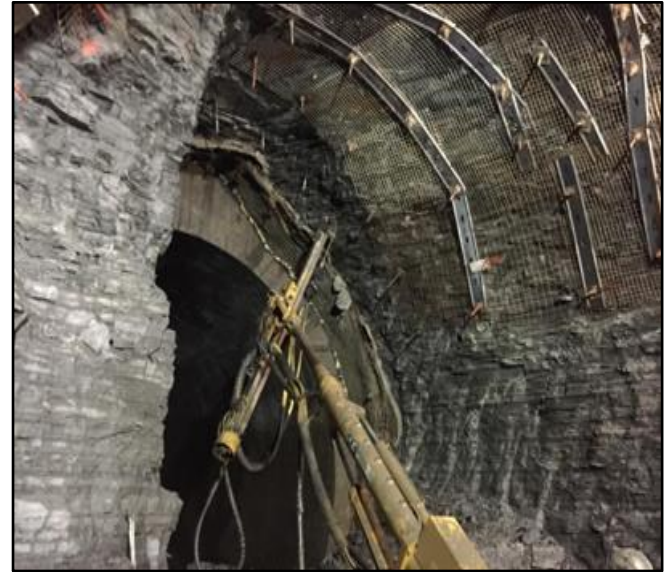
Fig 5 Tunnel Stabilization in Progress
