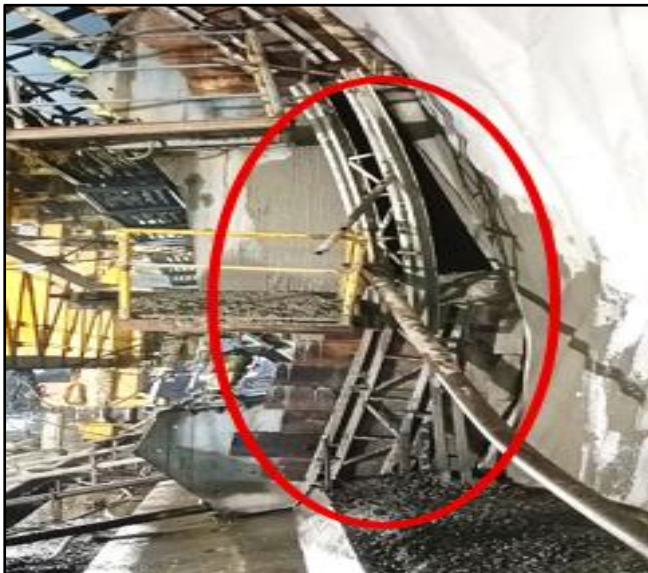
Fig 8 Bulk End Failure
