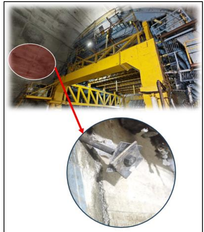
Fig 7 Indicating Uneven (Stepping) Surface of Concrete Due to Panel Discontinuity
