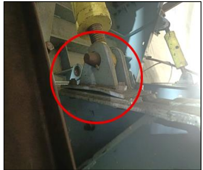
Fig 9 Indicating Failure of Plate Due to Differential Settlement
