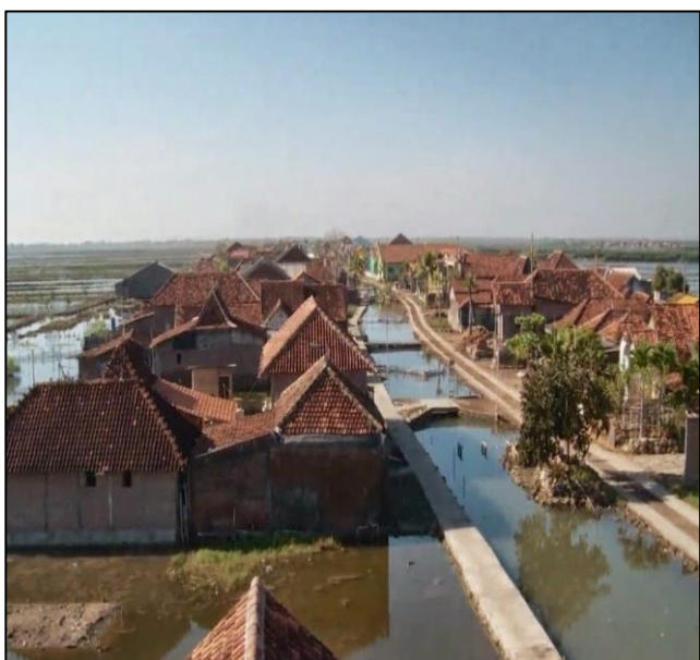
Fig 2: Condition of Timbulsloko
