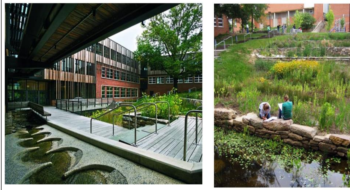
Fig 4 Constructed Wetlands and Outdoor Learning Spaces at Sidwell Friends Middle School, www.asla.org
