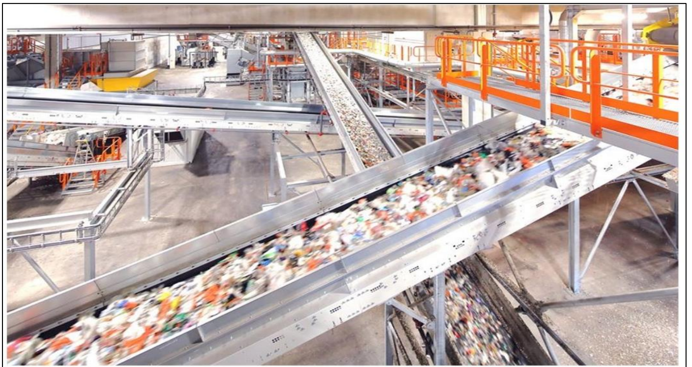
Fig 10 Interior View of Site Zero, Motala. Source: (HEBDO CONSTRUCTION, 2022b)
