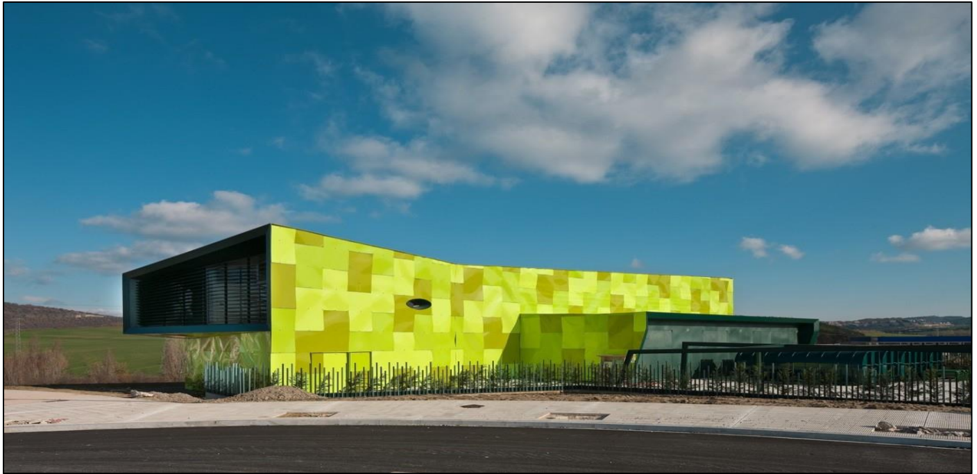
Fig 5 Exterior View of Urban Solid Waste Collection Central
