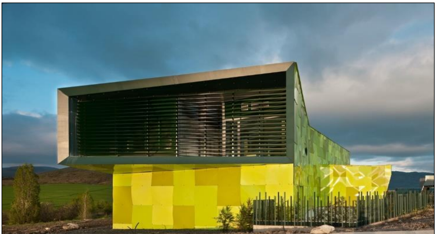
Fig 8 Exterior View of Urban Solid Waste Collection Central
