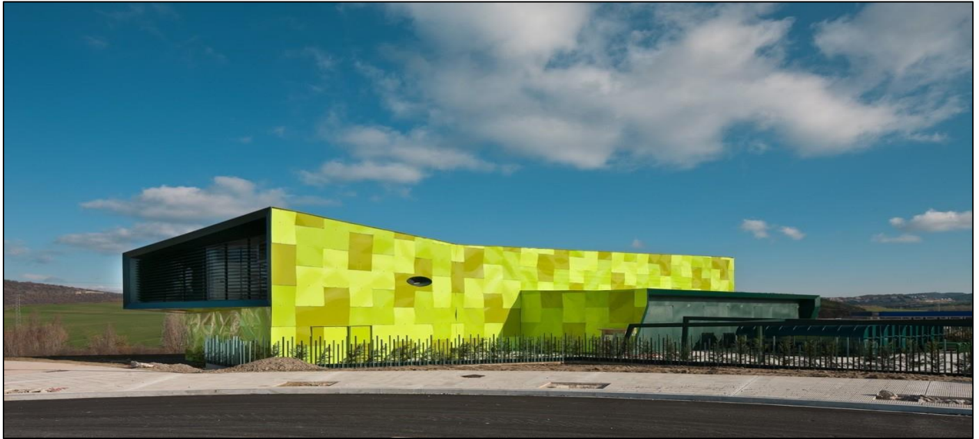
Fig 9 Exterior View of Urban Solid Waste Collection Central
