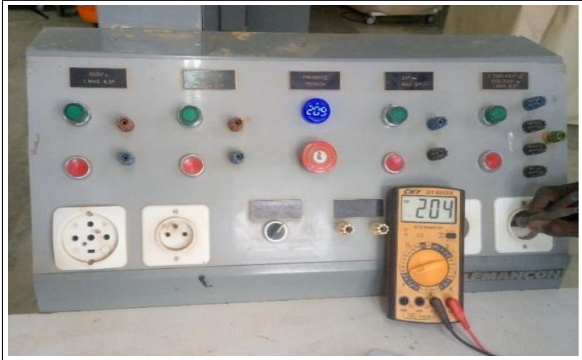
Voltage Measurement in the Socket Circuits
