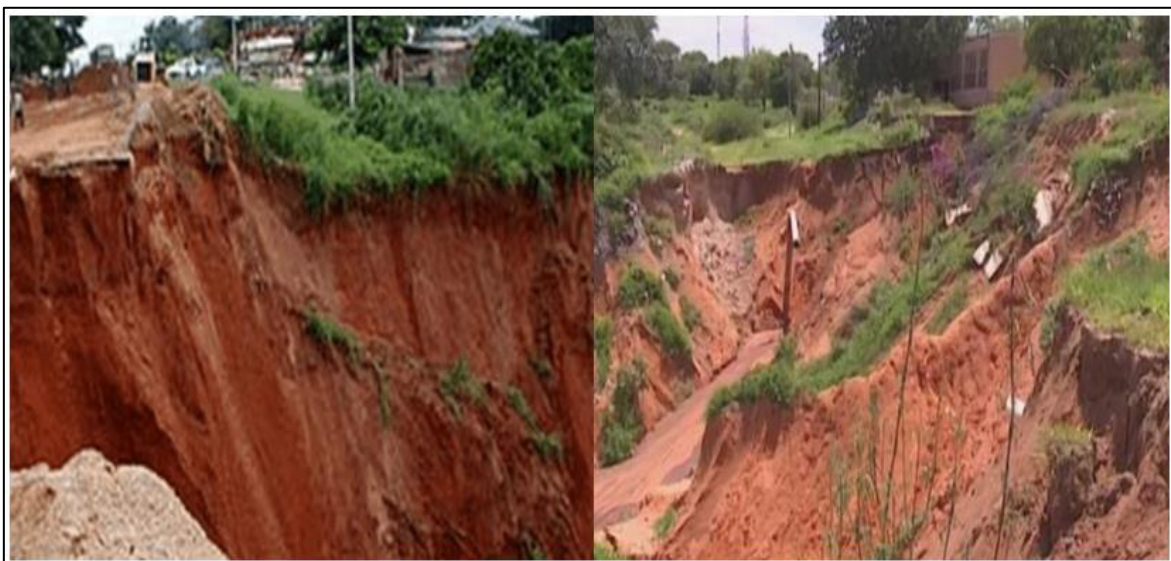
Plate 2 Photos of Eroded Areas
